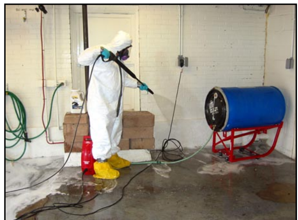
Figure 2. Using a pressure washer to clean contaminated surfaces.
