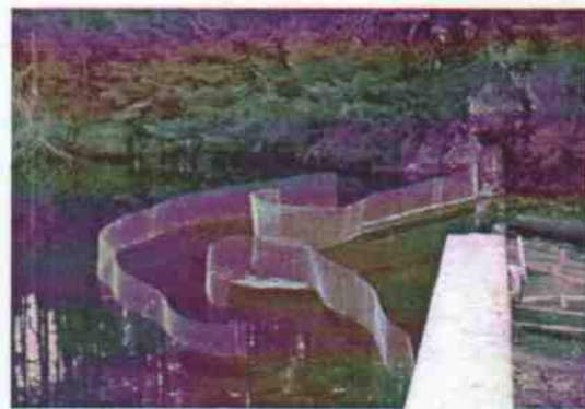
Deflector and collector screens in front of an inclined screen trap
